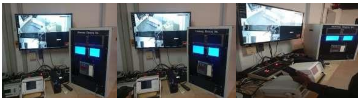
Plate 3: Control Room for Monitoring of Radiation Dosages and Timing
